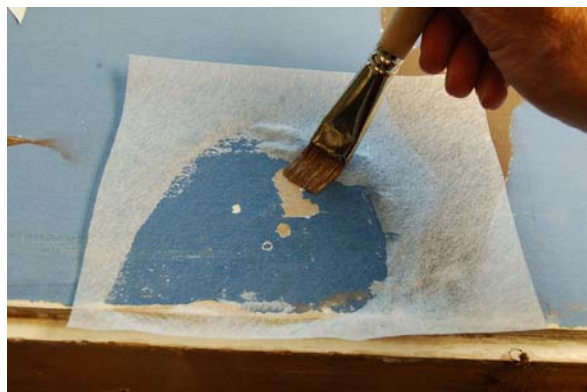
Figure 7 JunFunori is applied through a thin tissue.
