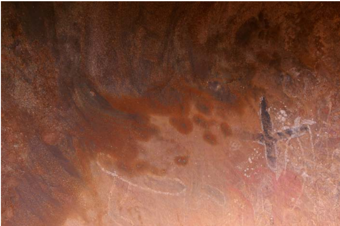
Figure 4 Identified need for consolidation in saline rock at Uluru. Desalination trials have preceded any discussion of consolidation. The areas to the top and right are darkened through water saturation with resultant spalling.
