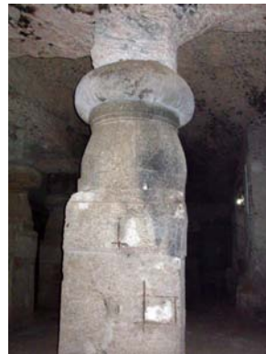
Figure 6: Corrosion of steel within the repaired matrix gave rise to eventual issues of splitting and spalling
